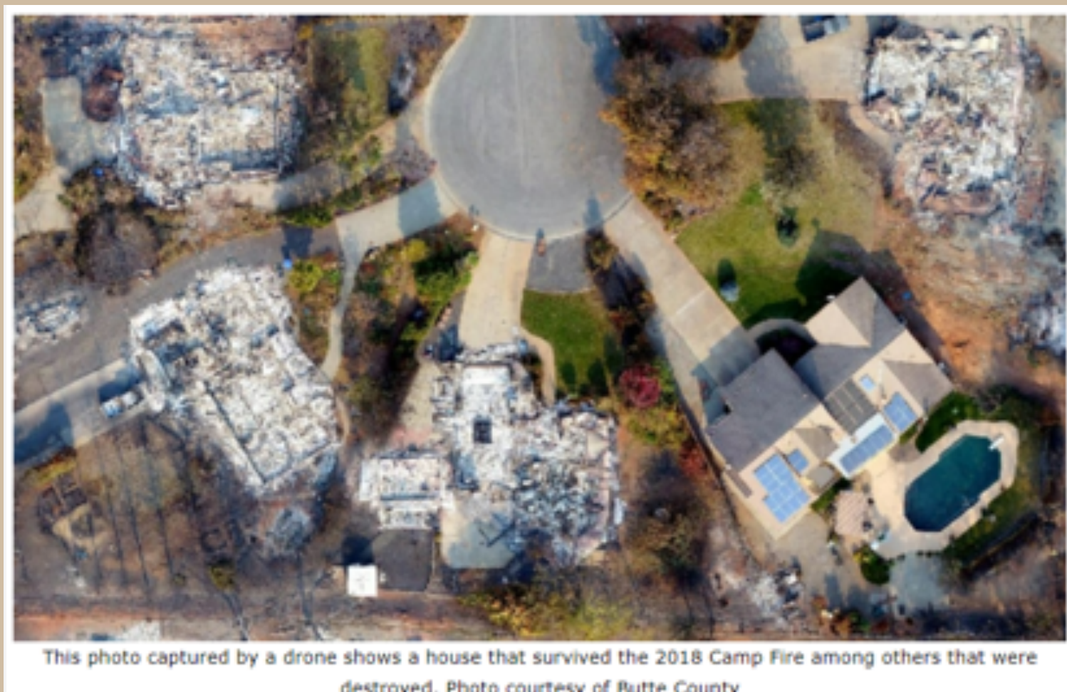
This photo captured by a drone shows a house that survived the 2018 Camp Fire among others that were destroyed. Photo courtesy of Butte County
